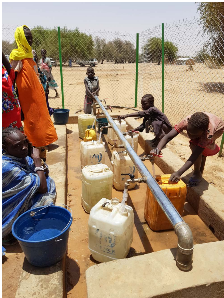
The positive impact of SDC’s WASH expert Walter Baumgartner, who was working for UNHCR’s WASH response. As a very tangible result of his secondment, all refugees in the camp had access to sufficient water, and the latrine situation was improved. El-Nimir camp East Darfur, Ed Daein, May 2018
