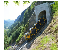
The Stoosbahn is the steepest funicular railway in the world, reaching a gradient of 47 degrees © Switzerland Tourism
